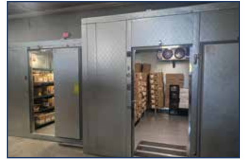
New walk-in freezer (right) for frozen food and meats and walk-in cooler (left) for fresh produce and dairy products Photo credit: Katie Draeger
